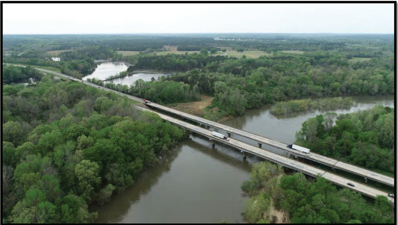
A view of the western bank of the Wateree River.
