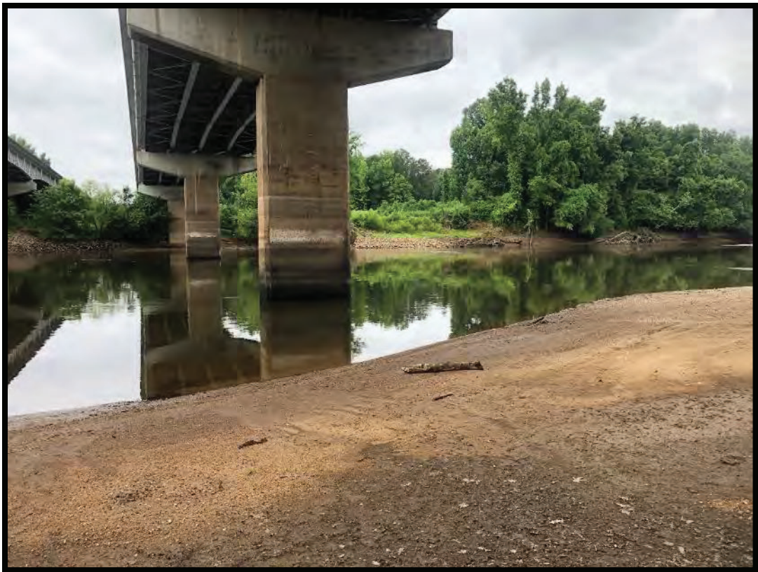
Westbound I-20 bridge (facing southwest).
