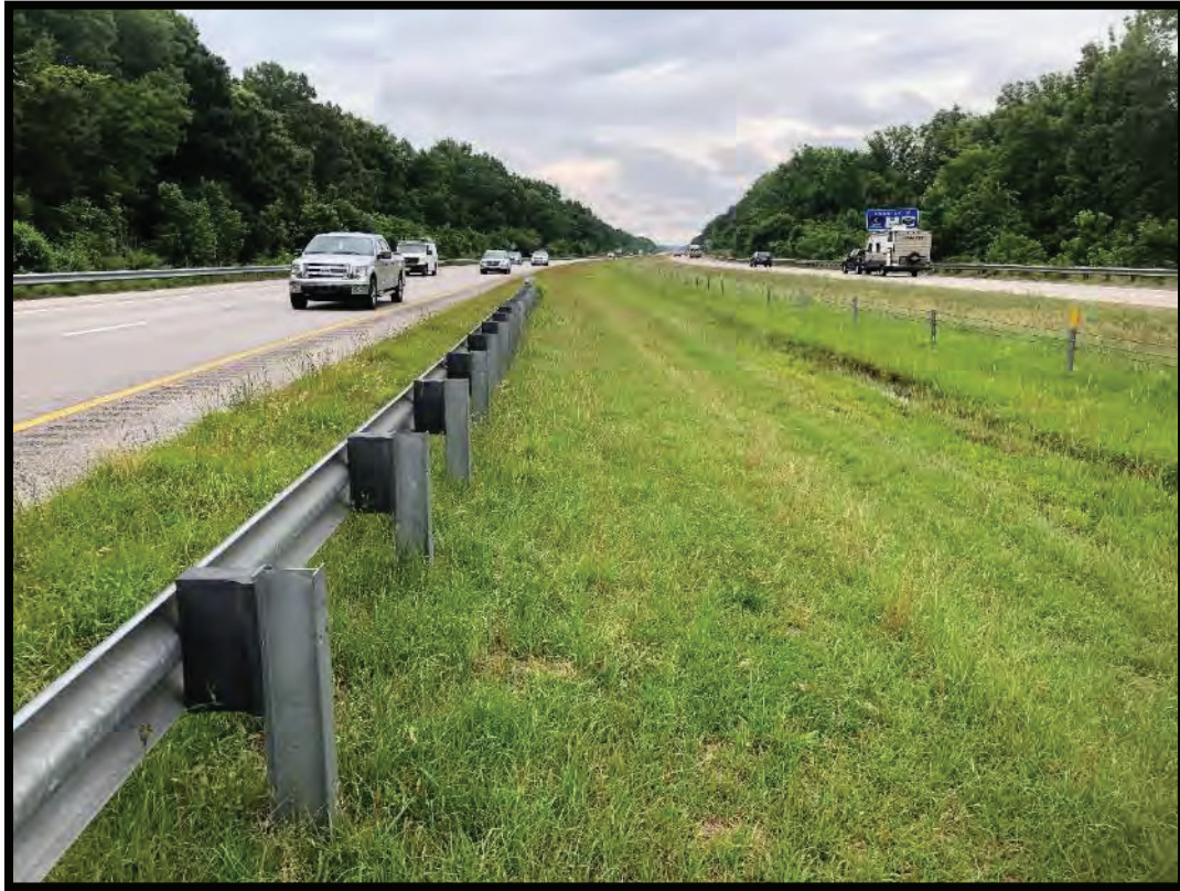
Typical maintained medians.
