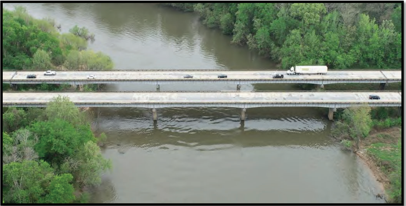
A view of the existing I-20 bridges facing south southeast.
