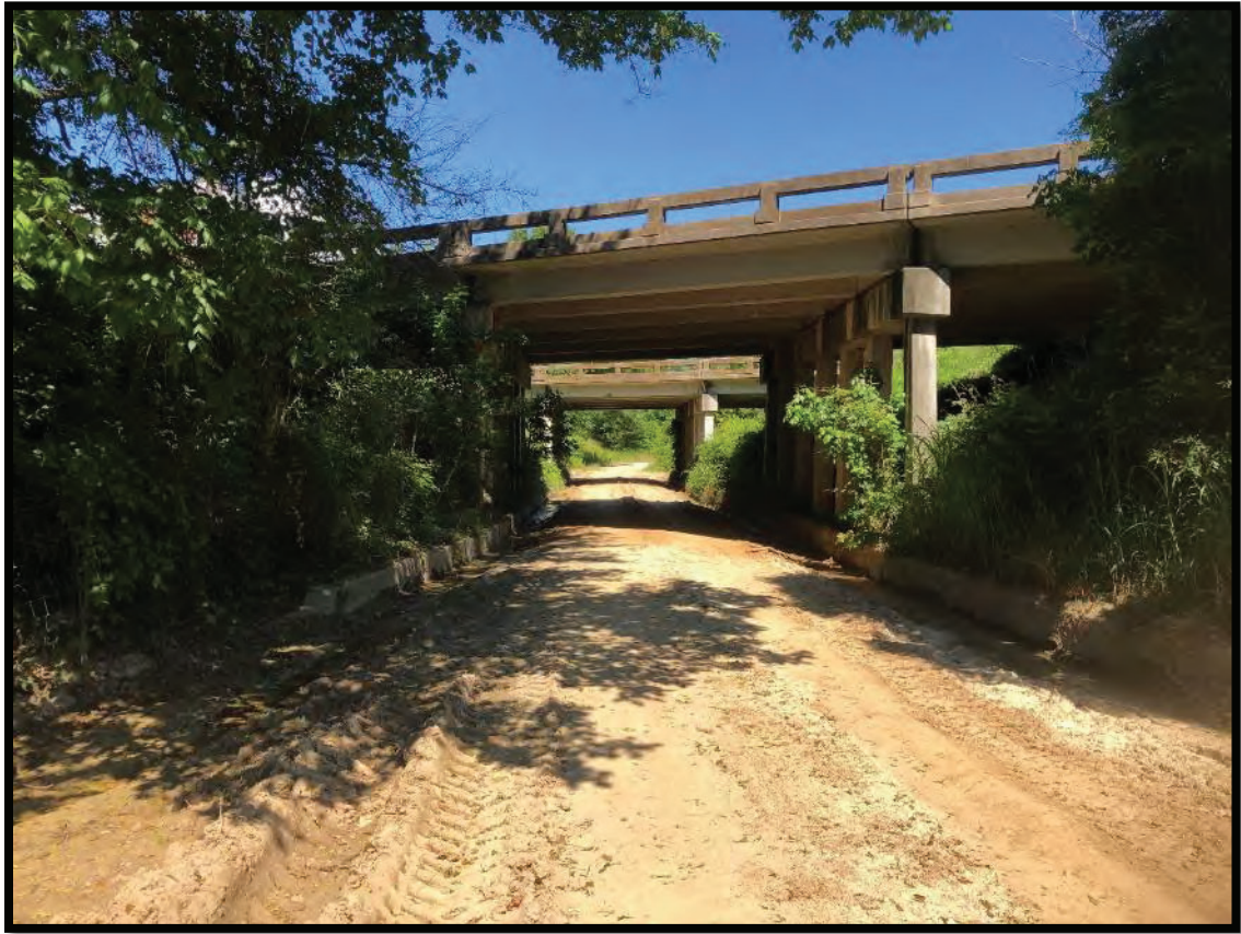
Bridges over dirt access road.
