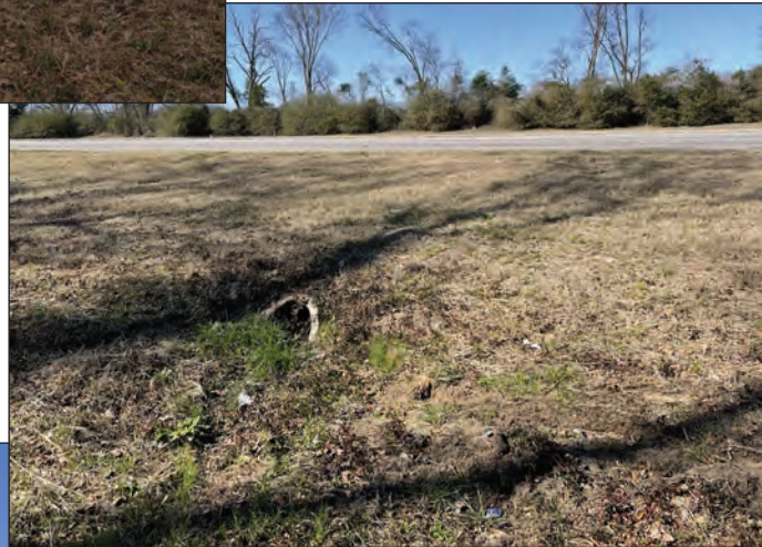
b. Drain Outlet Shown on Engineer's Drawing, Facing North
