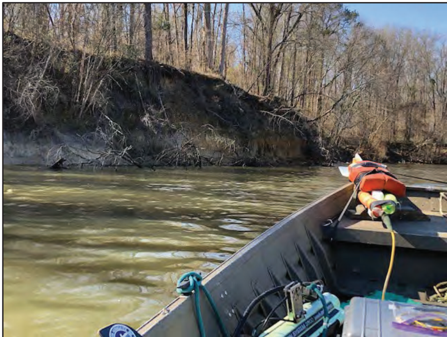
Plate 4. View of the Western Shoreline, Upstream of I-20 Bridges. Photographer: Ralph Wilbanks; Date: February 01, 2022)
