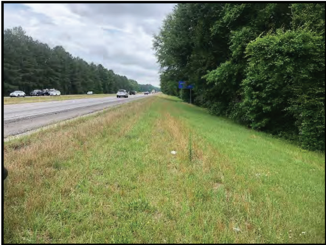
Typical maintained road shoulders.
