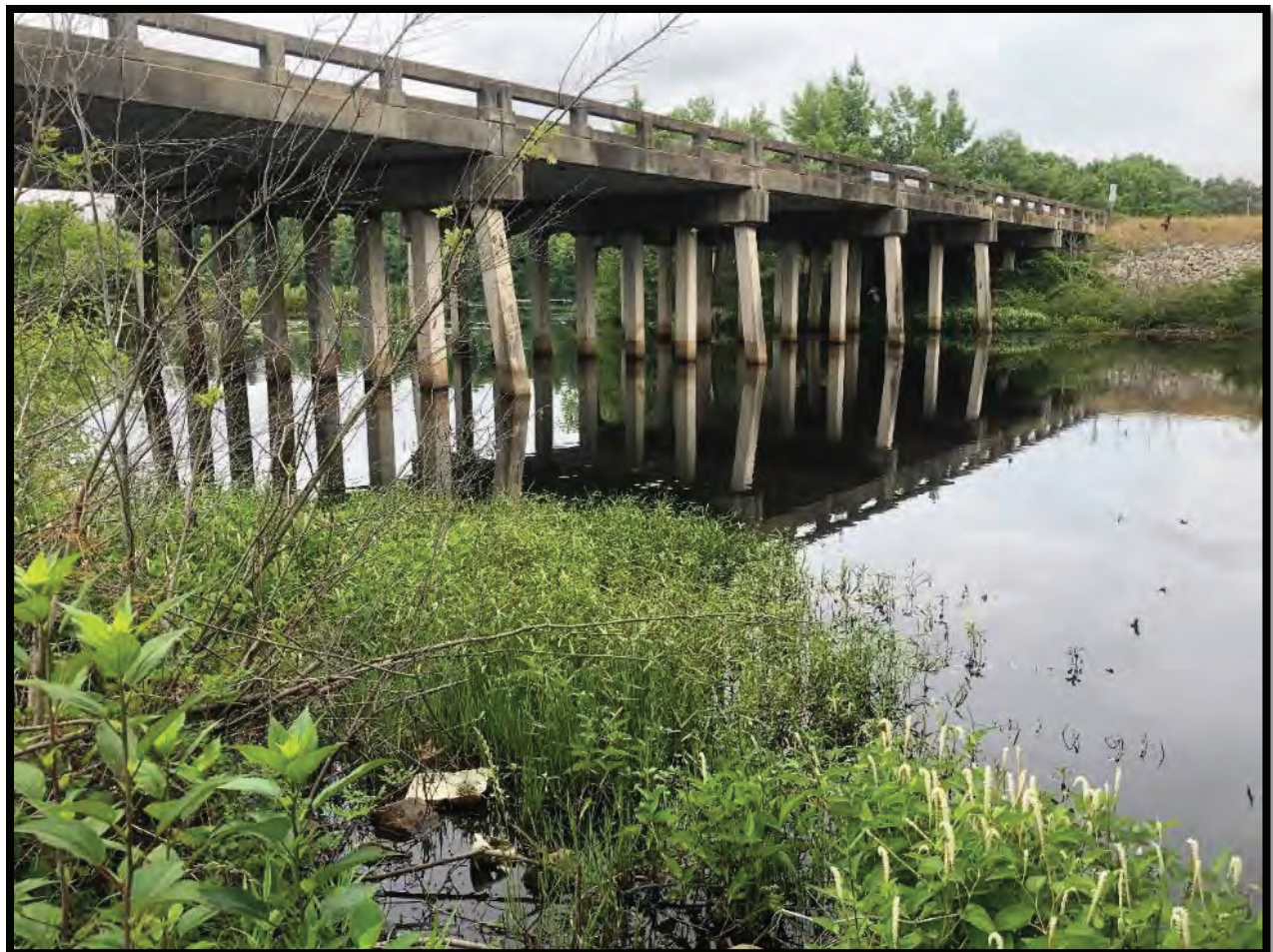
Westbound bridge over Buck and Gillies Creeks impoundment.
