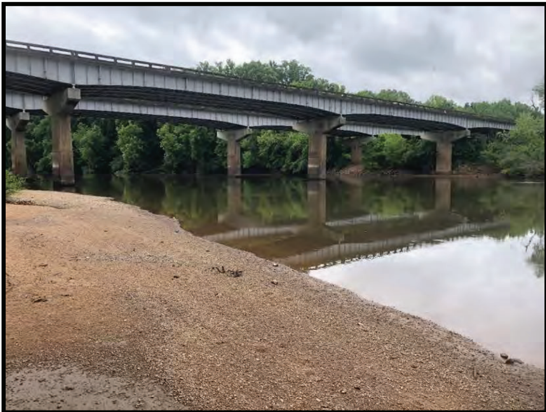
Wateree River bridges.
