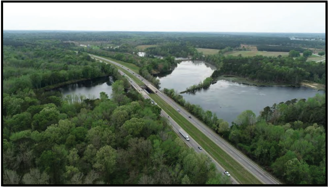
Ponds constructed in Buck and Gillies Creeks, west of the Wateree River.
