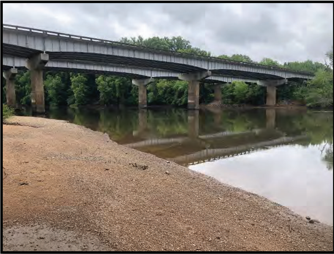
Existing I-20 bridge piers (facing south).
