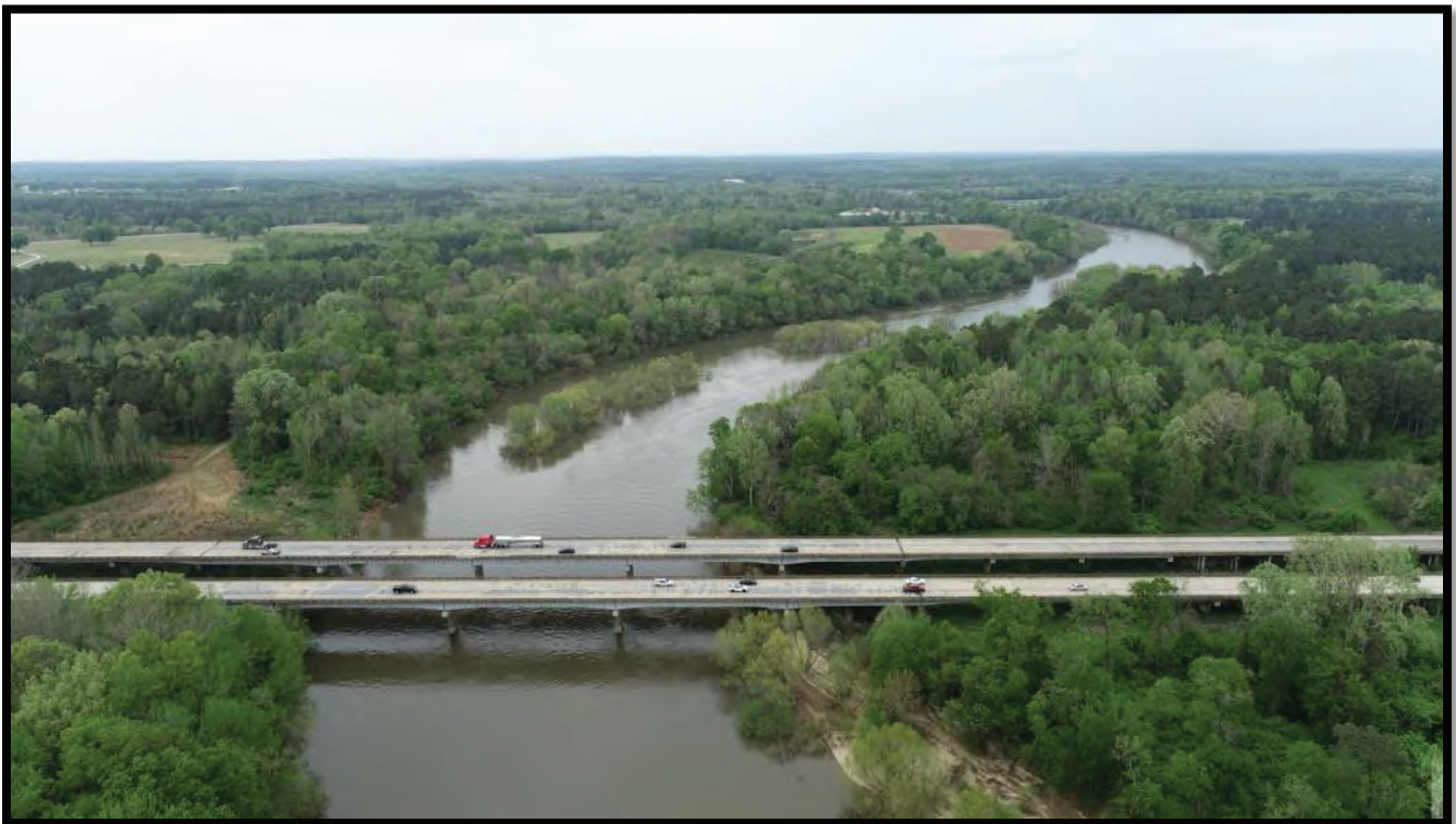
A view of the existing I-20 bridges facing north northeast.
