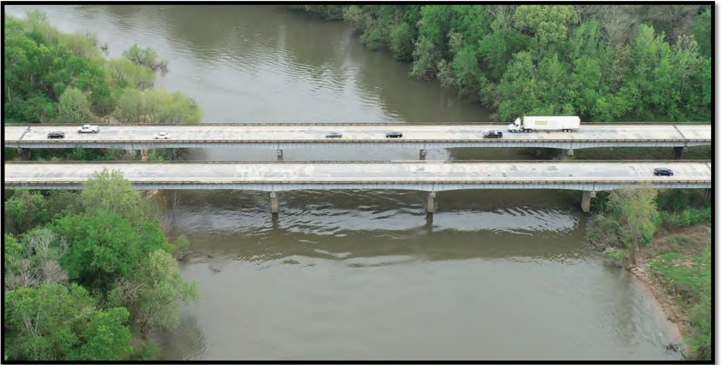
Existing bridge structures in the Wateree River.
