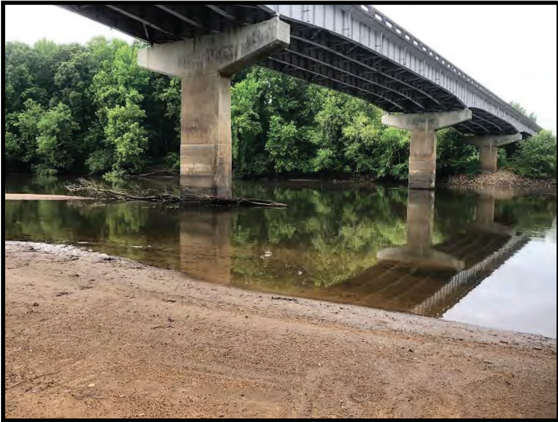
Eastbound I-20 bridge (facing southwest).
